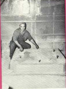
A new hoist was installed in the shipping department. Oren Gowers kneels by the cement slab to which the hoist will be fastened.
