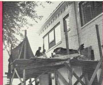
Repairs were made. Workmen are laying bricks on the entrance to the office building.
