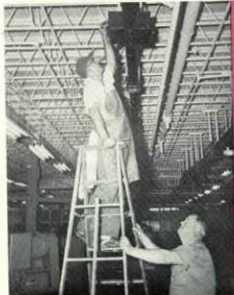
Hillard Garner turns off the current before beginning to work on a machine. The ladder is being attended by Hugh Arnold. Safety is important at all times whether during regular working hours, or not.
